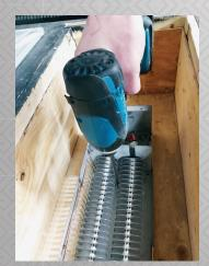
Use the 2 fixing holes in the bottom of the heater to secure it using appropriate screws (not supplied).
